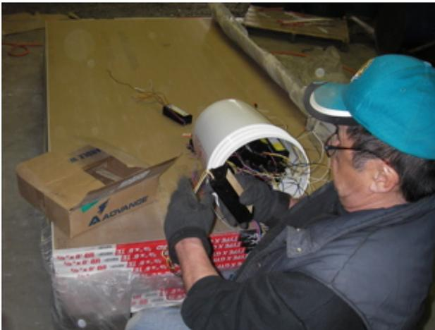
Double checking ballasts for PCBs
