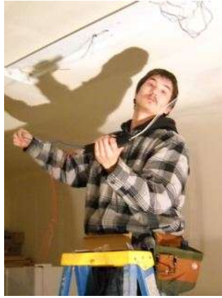
Maintenance Staff Charlie Doty retrofitting a 2-lamp fixture
