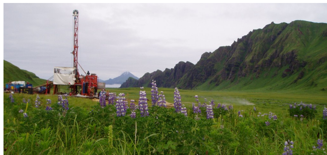
Geothermal resource assessment at Akutan.
