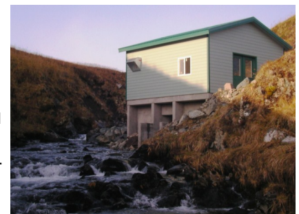
Powerhouse for Atka hydro project.
