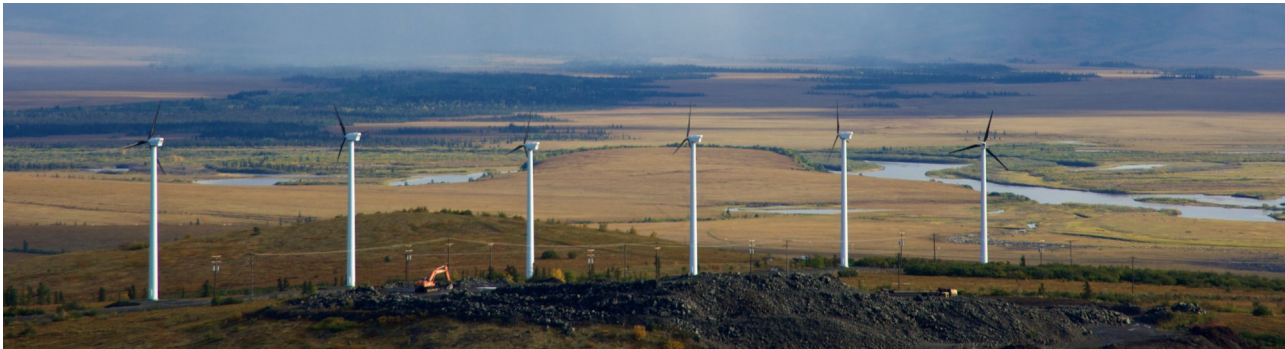
Six Unalakleet wind turbines.
