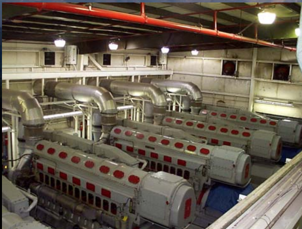
UniSea Inc. uses over one million gallons per year of 50-50 raw fish oil and diesel blend in their Unalaska power system.
