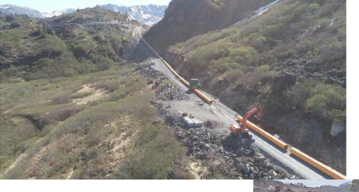
The project diverts runoff from Battle Creek into Bradley Lake expanding the state's largest hydroelectric facility
