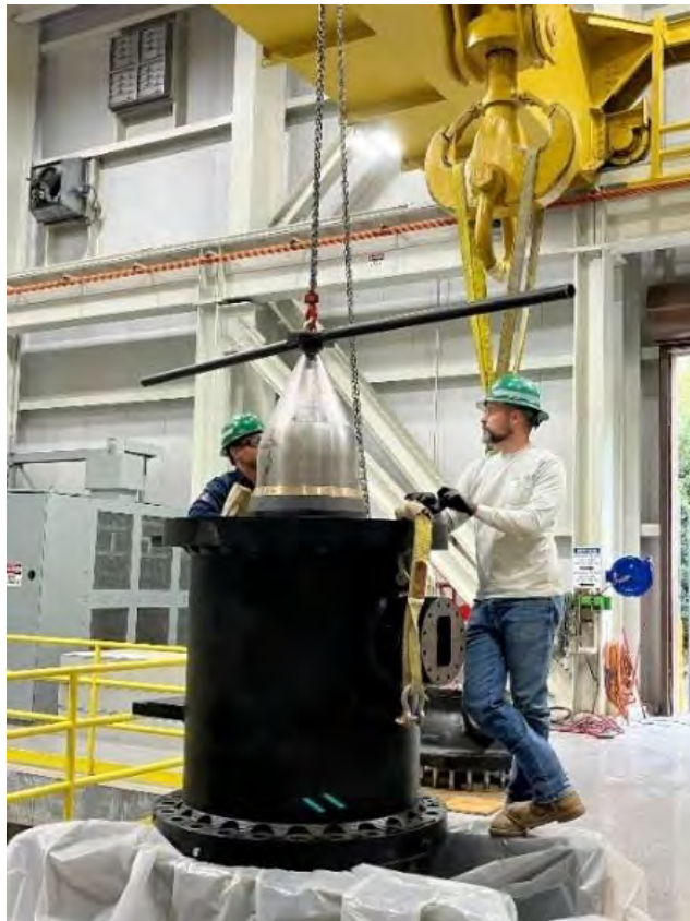
Removing the Needle Cone
