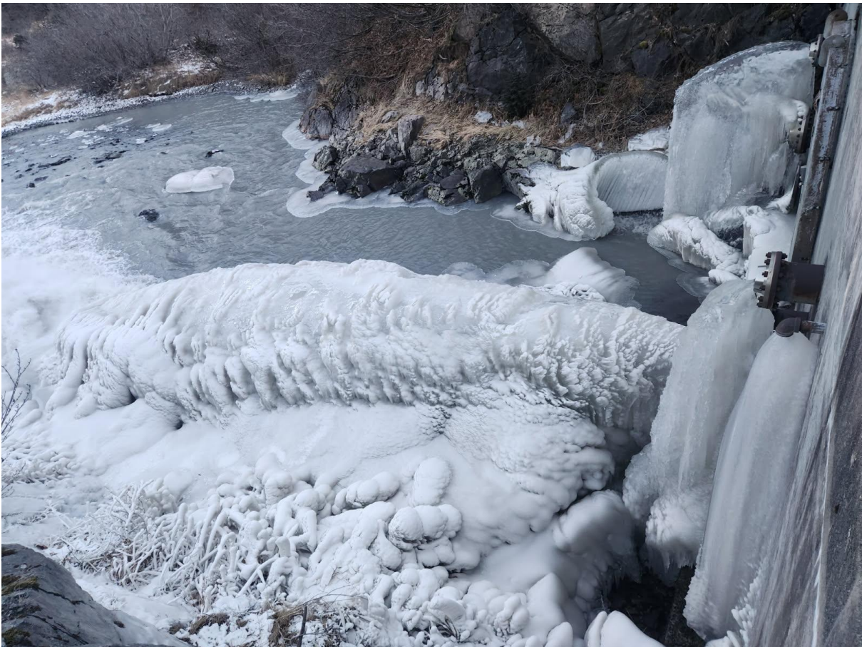
Ice Tunnel at the Fish Water Valves
