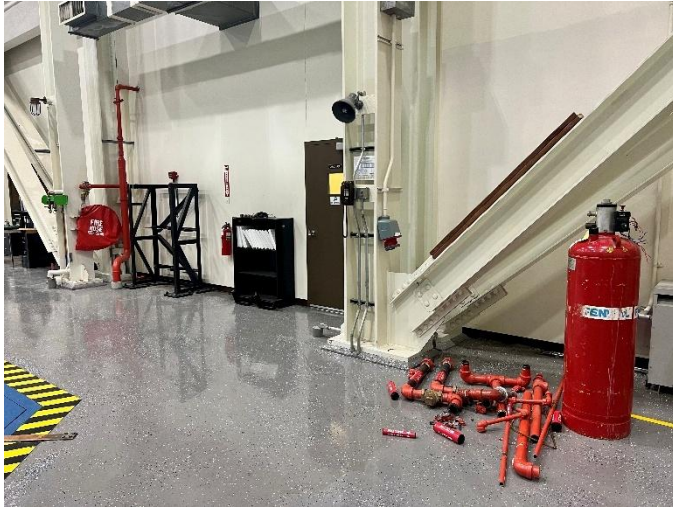
Removing the Halon Bottles
