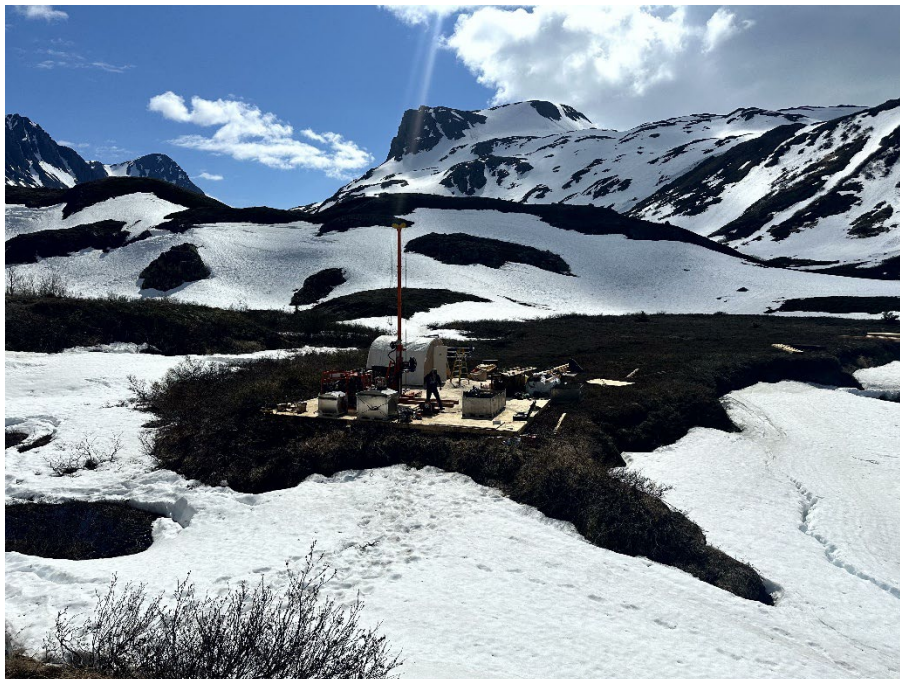
Tunnel Boring Alignment Drilling Platform
