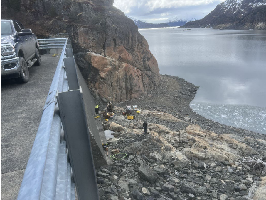
Frontside of Spillway Drilling
