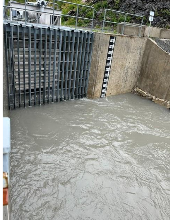
Battle Creek Diversion Pipe Inlet Pipe
