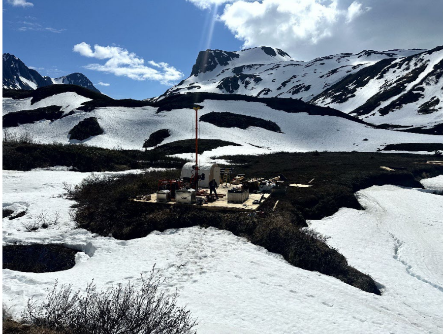
Tunnel Boring Alignment Drilling Platform
