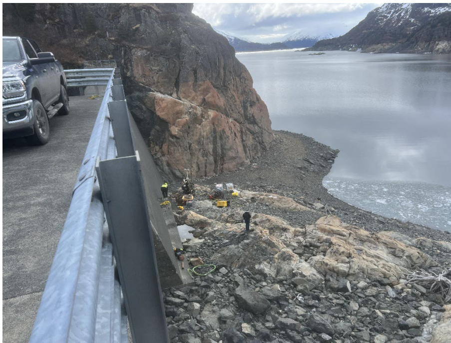
Frontside of Spillway Drilling
