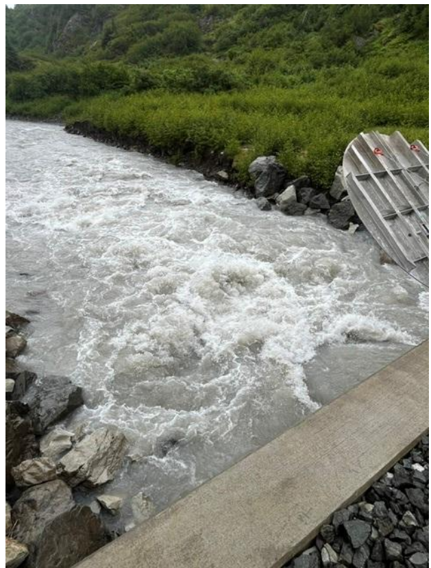
Battle Creek Diversion Pipe Outlet
