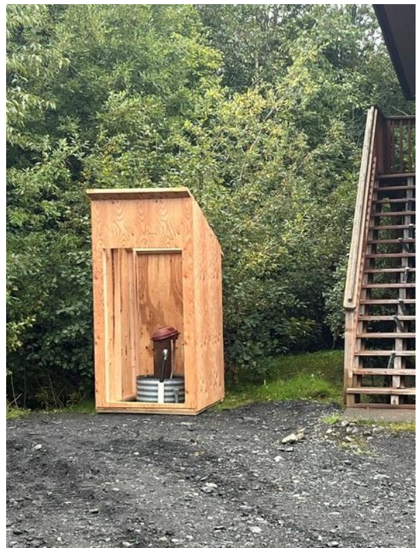
New Well House Under Construction
