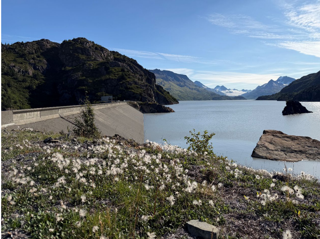
Bradley Lake Dam -September 1, 2026
